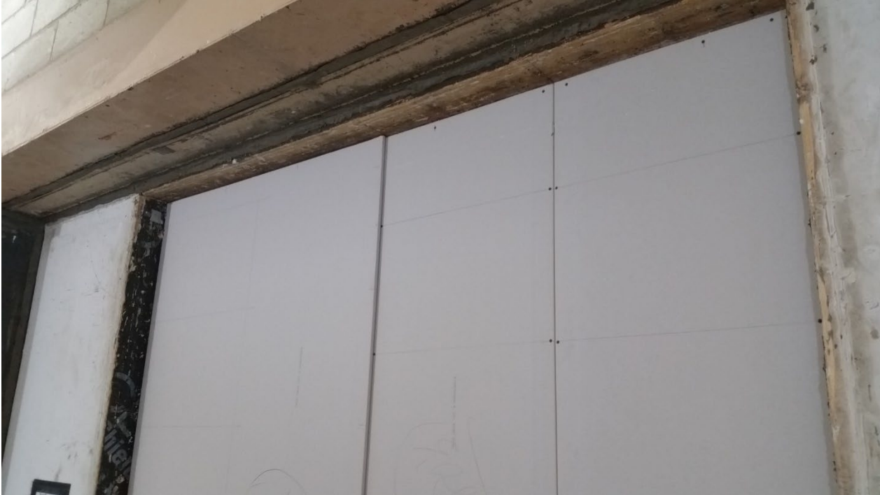
Figure 7 – Receive side base layer gypsum board installed, face layer gypsum board partially installed
