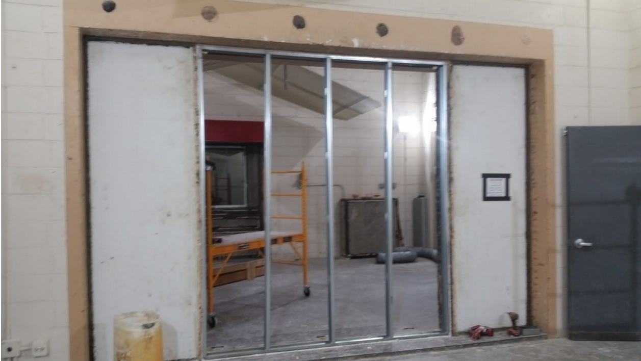
Figure 3 – Tracks and studs installed in test aperture
