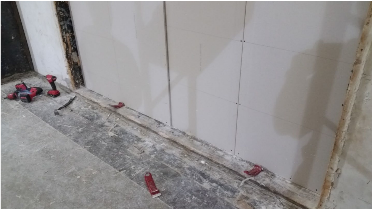
Figure 8 – Receive side base layer gypsum board installed, face layer gypsum board partially installed
