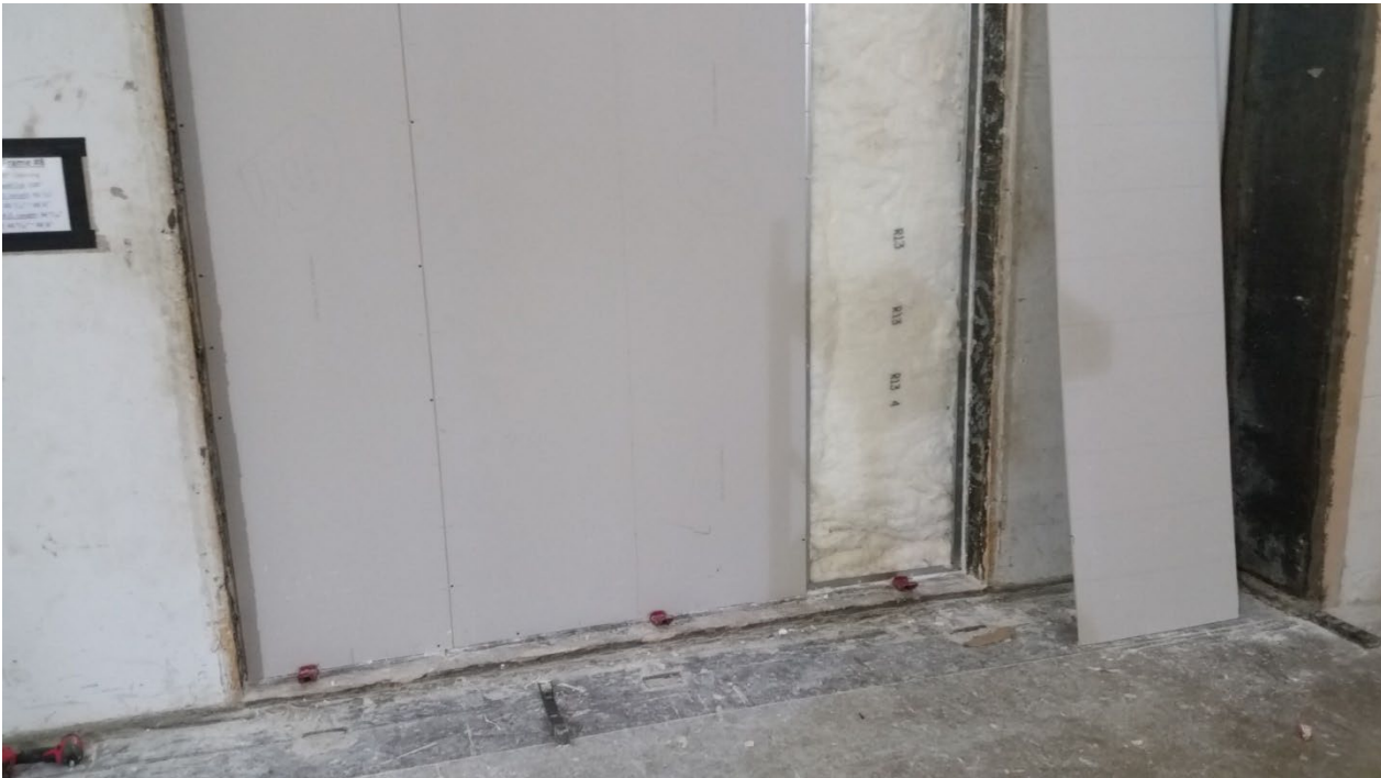
Figure 8 – Insulation installed in stud cavities, receive room side partially installed, viewed from receive room
