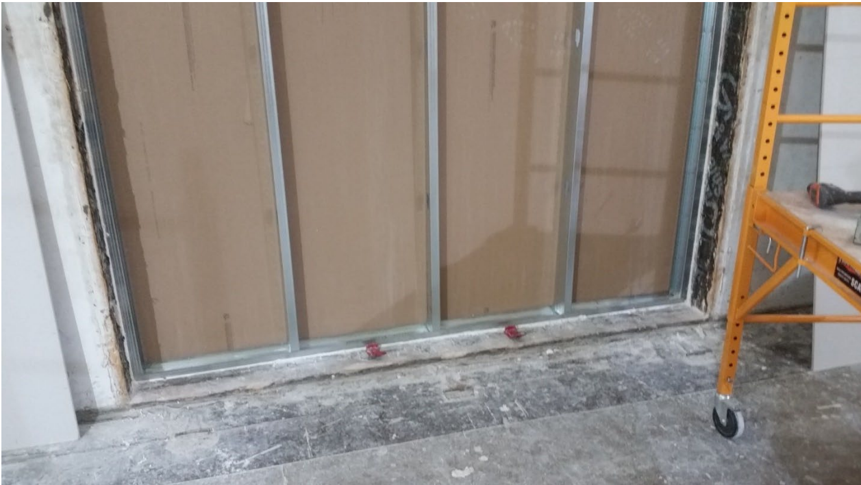
Figure 6 – Source room side gypsum board installed, viewed from receive room
