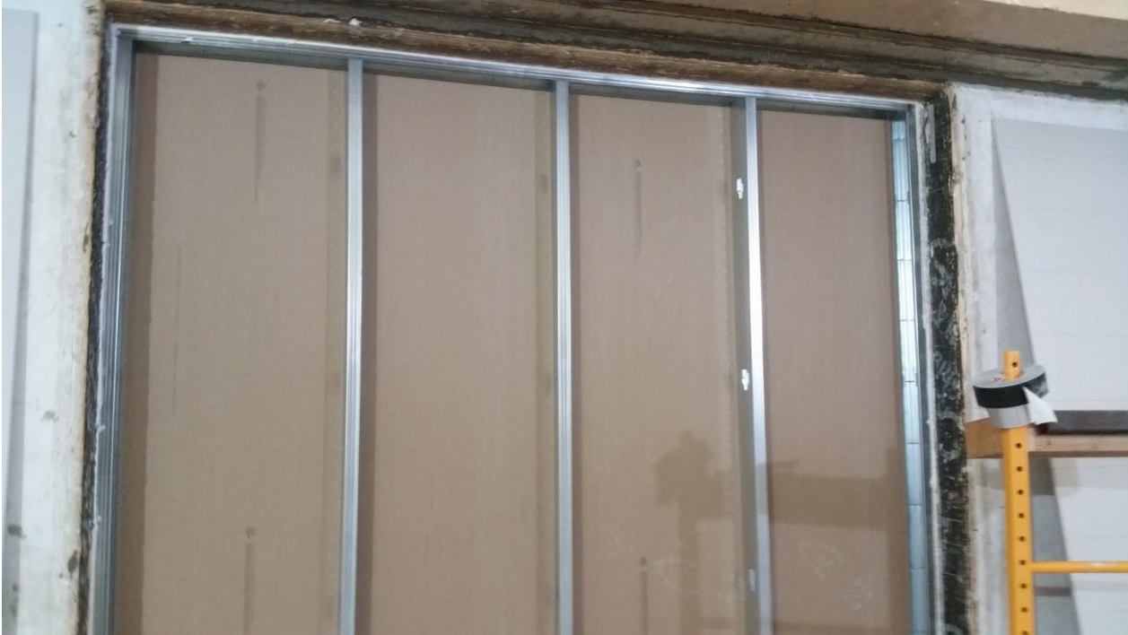
Figure 5 – Source room side gypsum board installed, viewed from receive room
