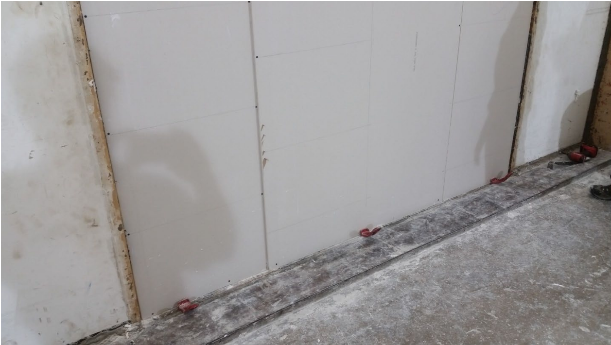
Figure 7 – Source room side face layer gypsum board partially installed
