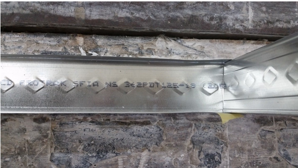
Figure 4 – Detail of stud and track
