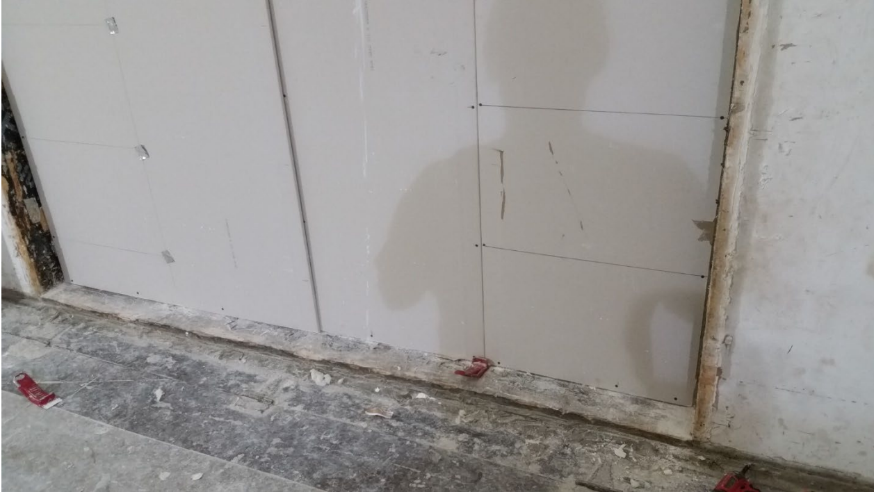
Figure 9 – Receive room side face layer gypsum board partially installed
