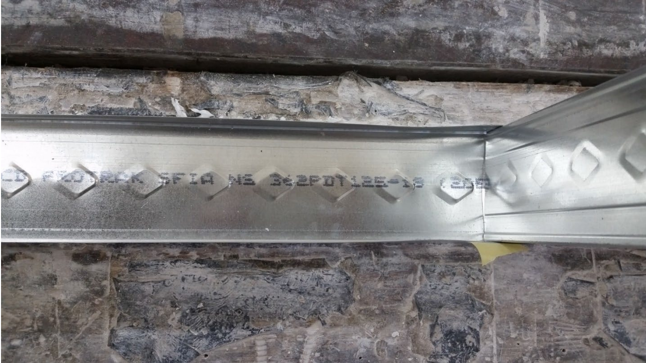
Figure 5 – Detail of stud and track
