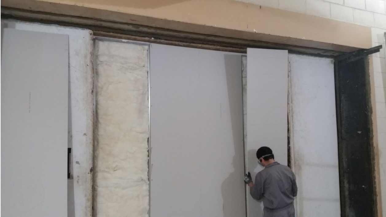
Figure 7 – Receive room side gypsum board partially installed
