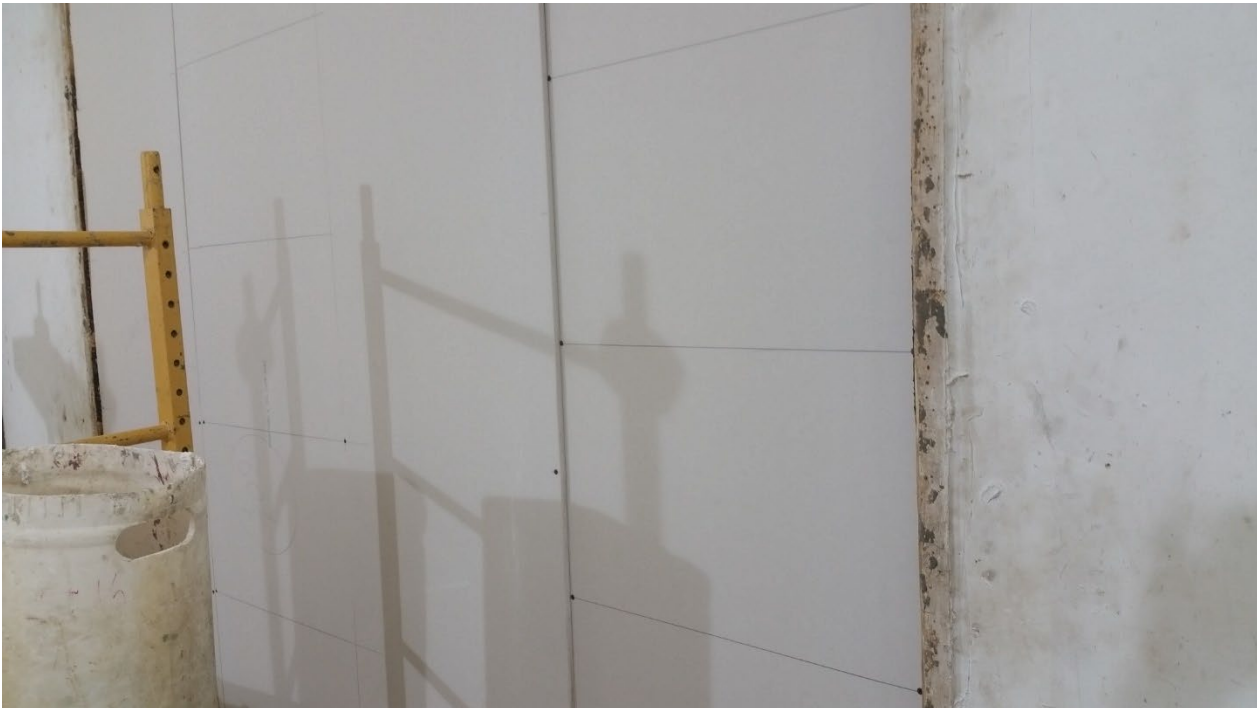
Figure 12 – Source side face layer gypsum board partially installed
