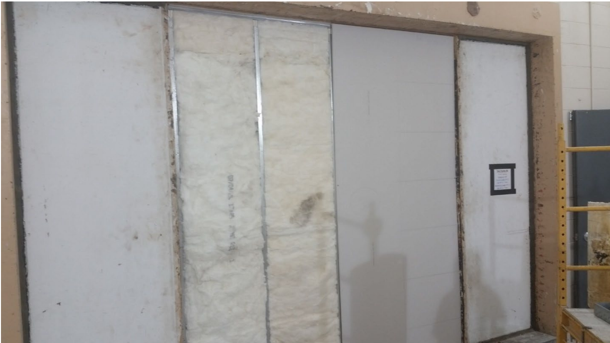
Figure 10 – Source side base layer gypsum board partially installed
