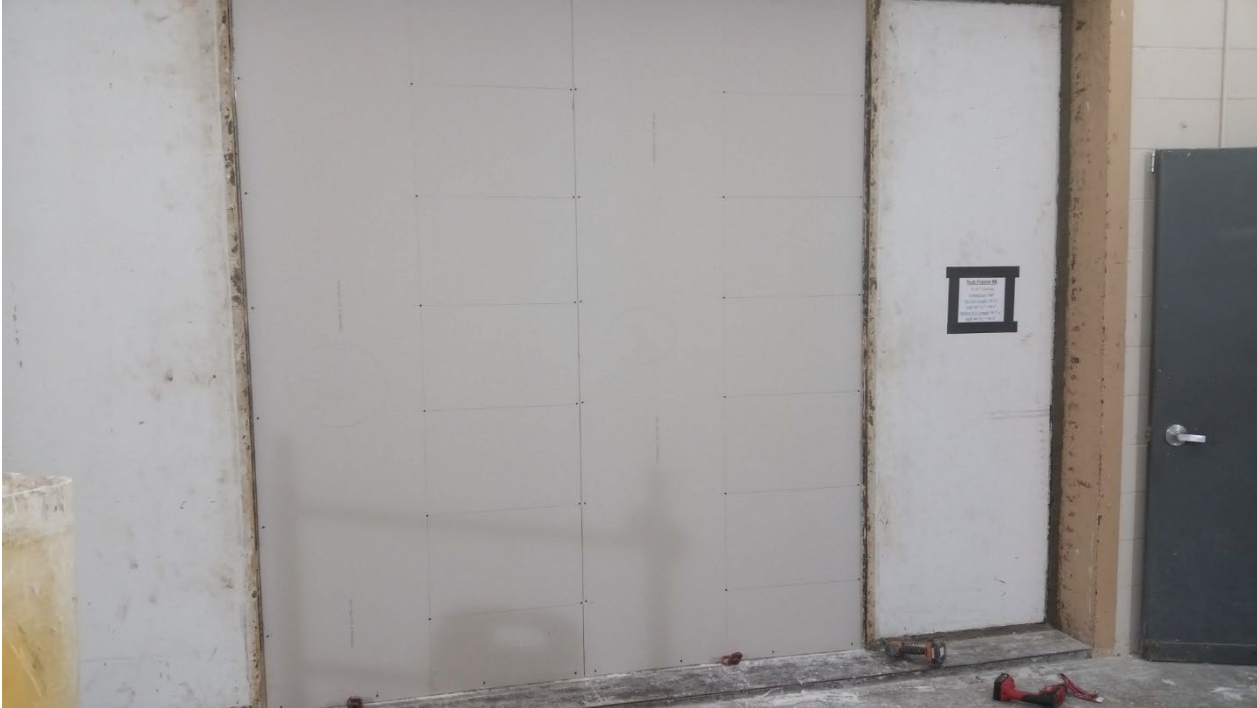
Figure 11 – Source side base layer gypsum board installed
