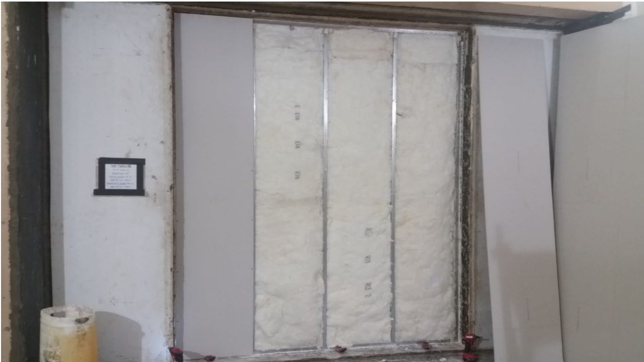
Figure 8 – Receive side base layer gypsum board partially installed
