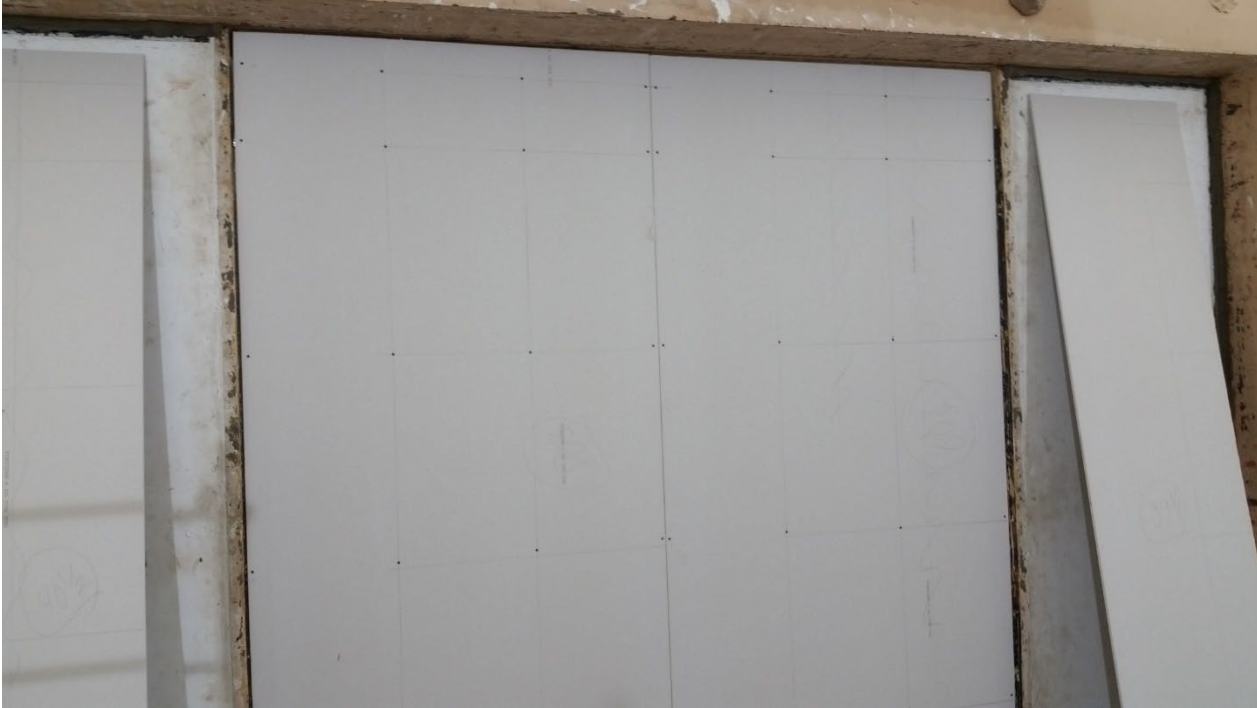
Figure 7 – Source side base layer gypsum board installed
