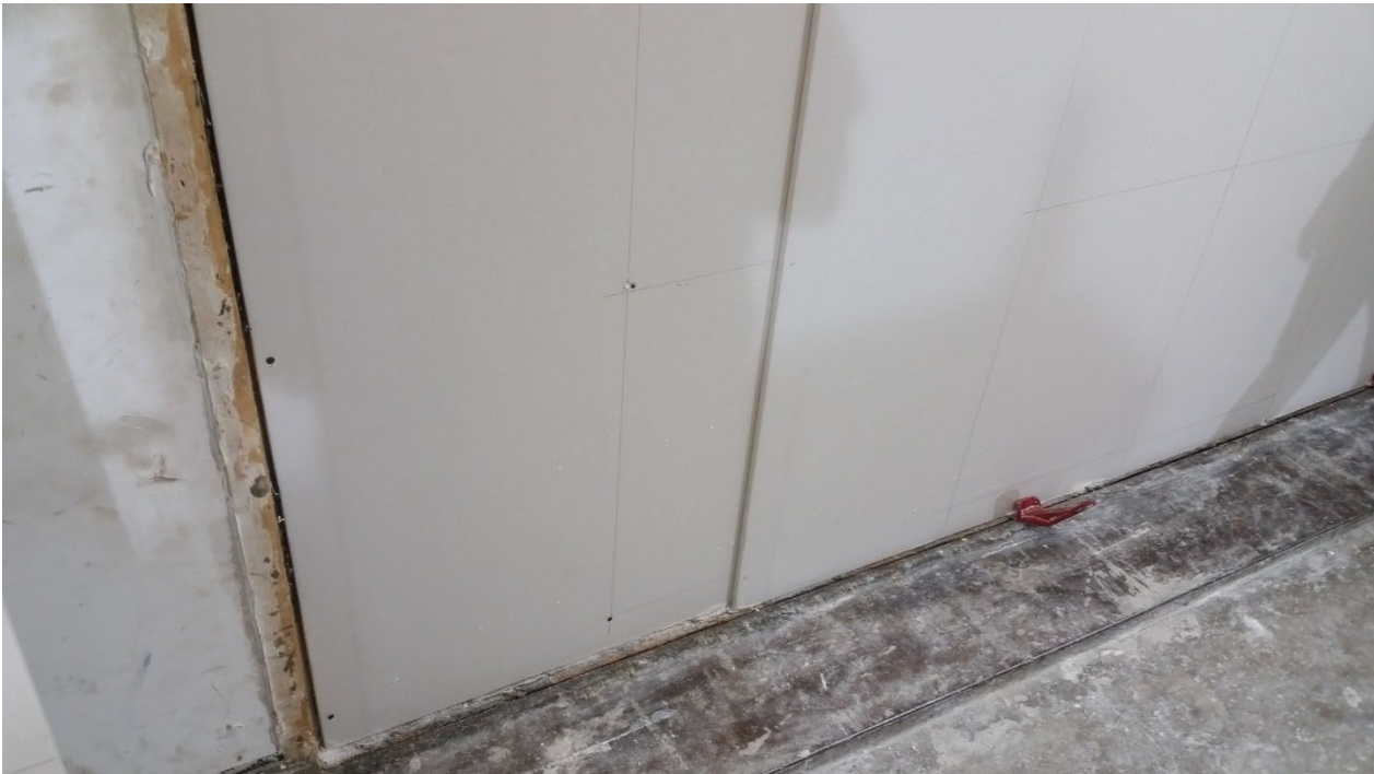
Figure 10 – Source side face layer gypsum board partially installed
