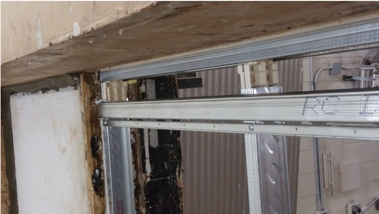
Figure 6 – Studs with ProStud Motion Frame Connectors fit into top track, resilient channel installed to source side of studs
