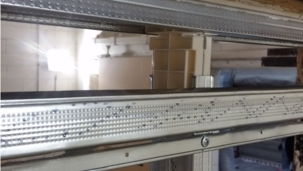
Figure 5 – Stud with ProStud Motion Frame Connector fit into top track, resilient channel installed to source side of studs
