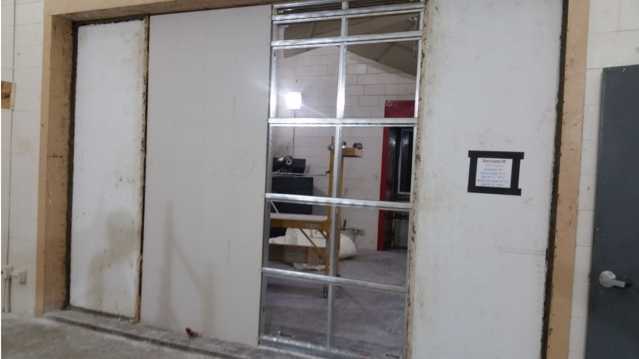
Figure 7 – Source side gypsum board partially installed
