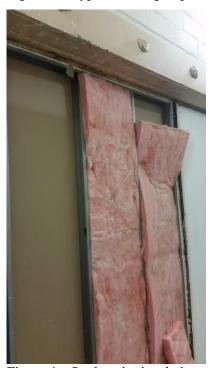
Figure 4 – Stud cavity insulation partially installed
