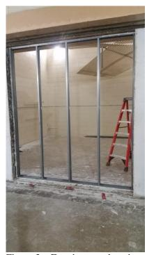
Figure 2 – Framing members installed in test aperture
