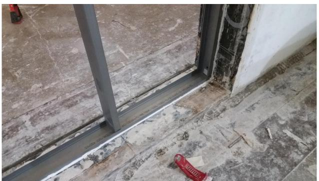
Figure 3 – Typical sealing of perimeter framing members, detail of floating stud
