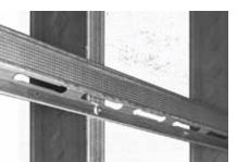
framing, with the elongated dog bone holes centered directly over the framing members. This placement helps impede airborne sound vibrations,
