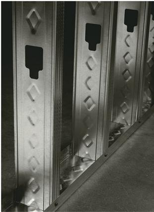
**WITH A HISTORY SPANNING MORE THAN HALF A CENTURY** in noncombustible commercial construction, cold-formed steel is a popular material choice for framing non-structural interior walls, load-bearing interior and exterior walls, floor joists, and curtain walls. The many performance-based characteristics and green attributes of cold-formed steel framing have enabled architects to design structures that are safer and more durable, dynamic as well as sustainable.
