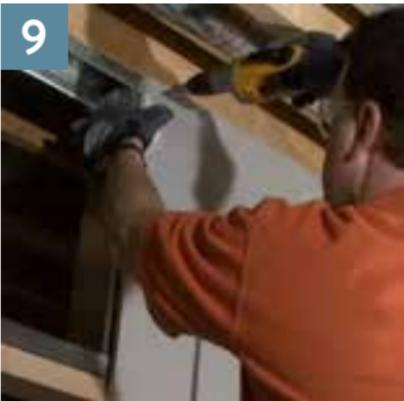
Attach drywall. Use corner bead around corners. Tape, spackle and finish drywall.
