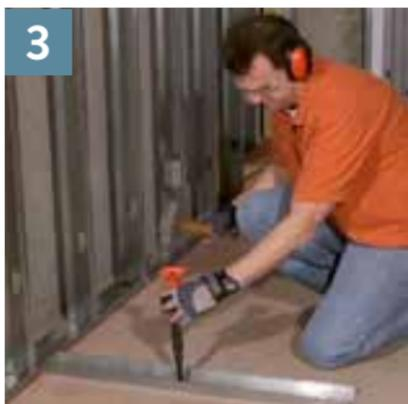
Attach floor runner using concrete anchors.
