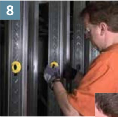
Snap in grommets for electric and plumbing.
