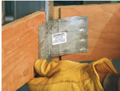
Flex Danback flexible wood backing around stud flange using the flexible connector plate.
