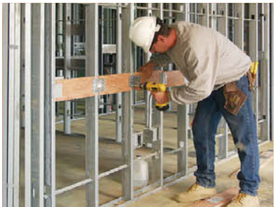
Secure each plate to the stud flange using two small pan or wafer head screws.
