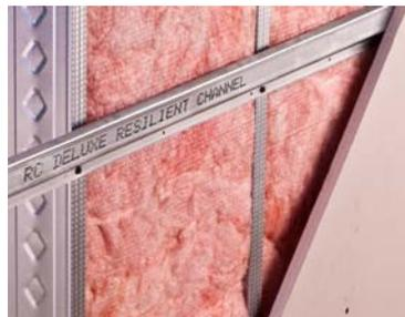
The first row of resilient channel, starting at the floor level, can be installed with the open side down to facilitate the connection of the resilient channel to the stud.
