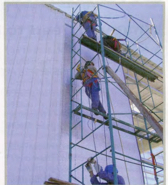
Fireproofing products help metal buildings obtain their hourly fire-resistance endurance ratings by withstanding fire impingement at a certain intensity for a specific amount of time. (Photo courtesy of RIMA International)
