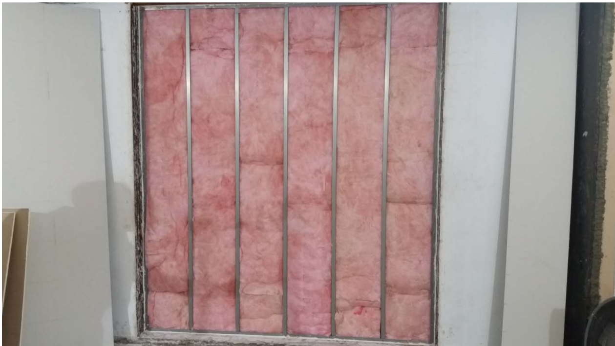
Figure 4 – Stud cavity insulation installed
