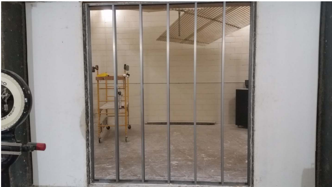
Figure 2 – Framing members installed in test frame aperture
