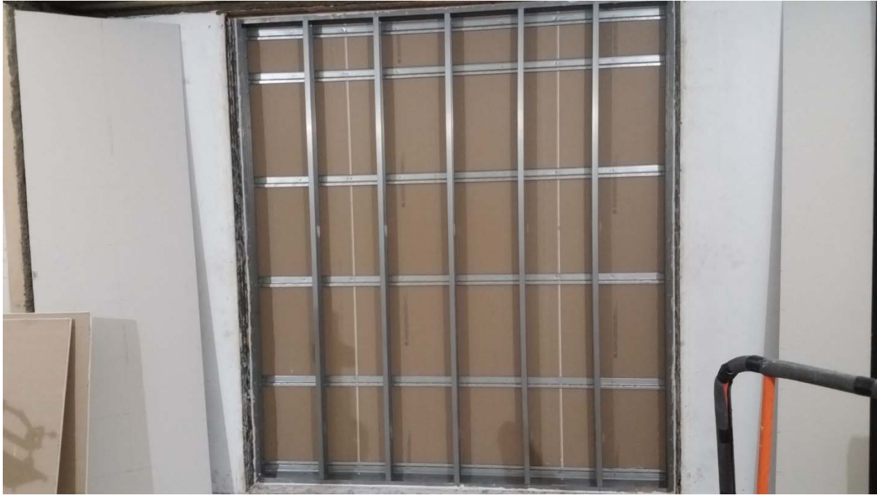
Figure 3 – Resilient channel and source side gypsum board layers installed, as viewed from receive room
