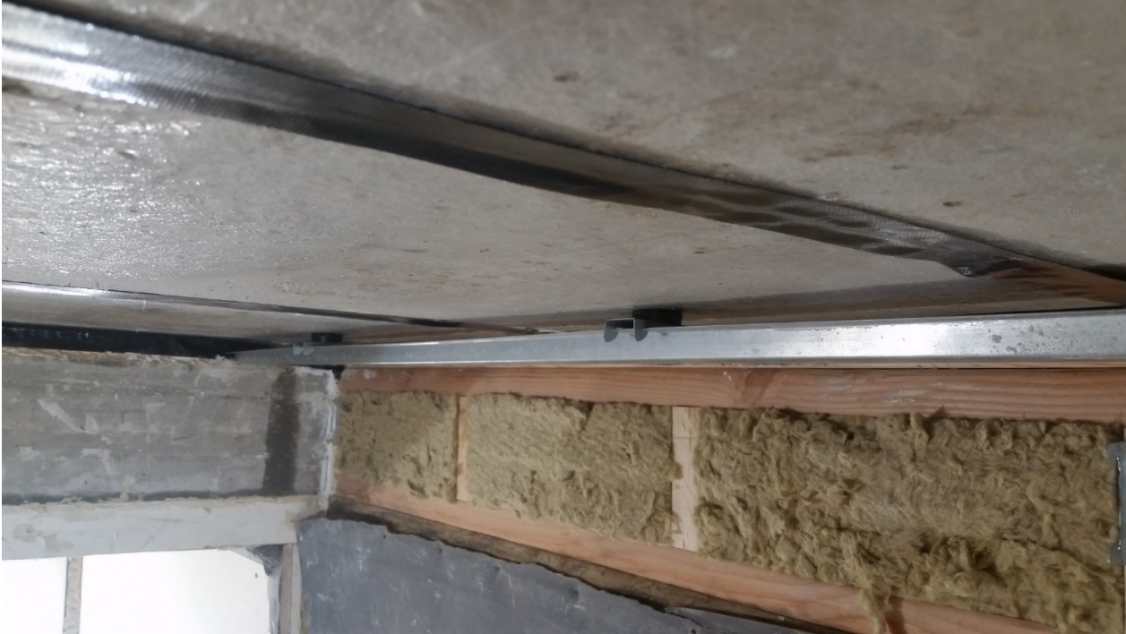
Figure 7 – Furring channel installed on isolating clips
