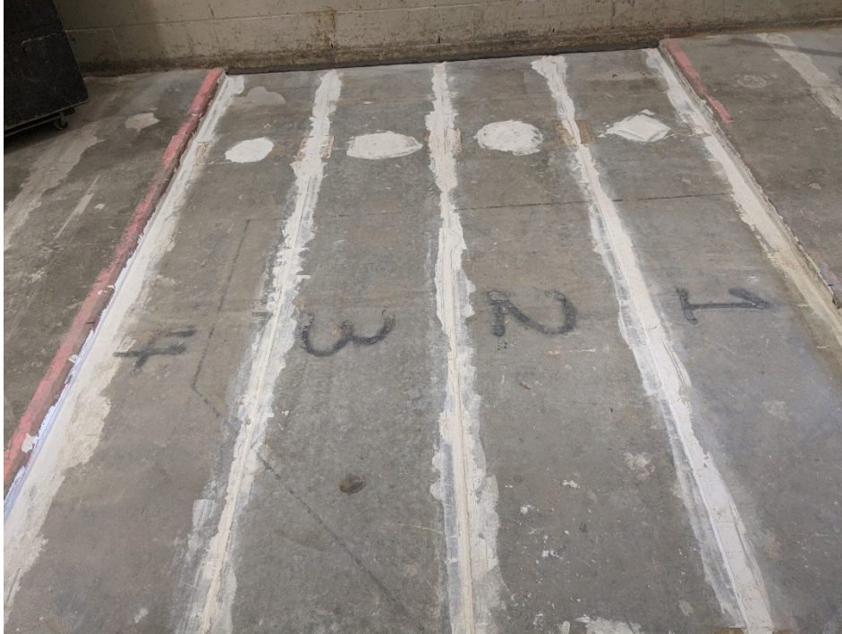
Figure 3 – Concrete slabs prior to installation of flooring, viewed from source room
