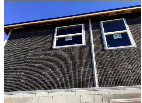
This is Welded Wire Lath (ASTM C933) with PVC accessories in the ClarkDietrich Lathing System called "Easy Embedment."
