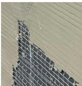
Welded wire lays down evenly with uniform furring.
