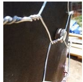
Woven wire often must be furred using nails to achieve the minimum required furring depth.
