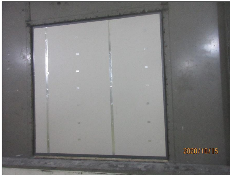
Photo No. 1 Receive Room View of Installed Specimen
