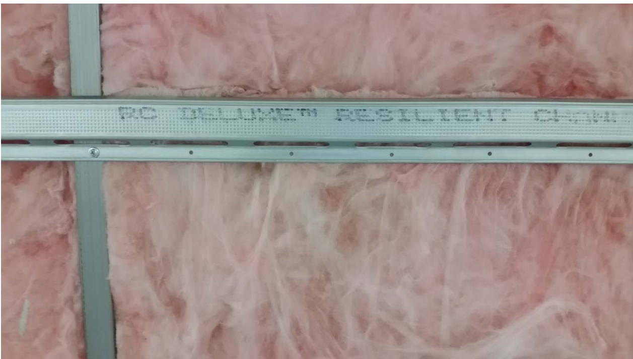
Figure 4 – Fastener placement, labeling on resilient channel
