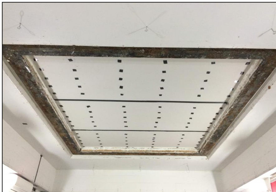
Photo No. 2 Receive Room View of Test Specimen Installation
