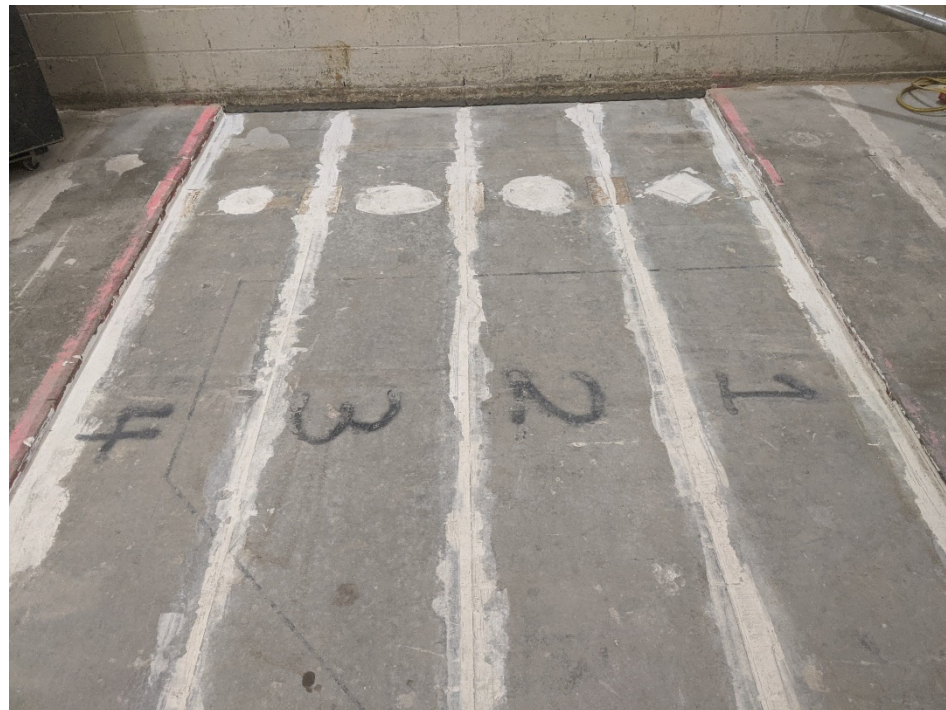
Figure 3 – Concrete slabs prior to installation of carpet flooring, viewed from source room
