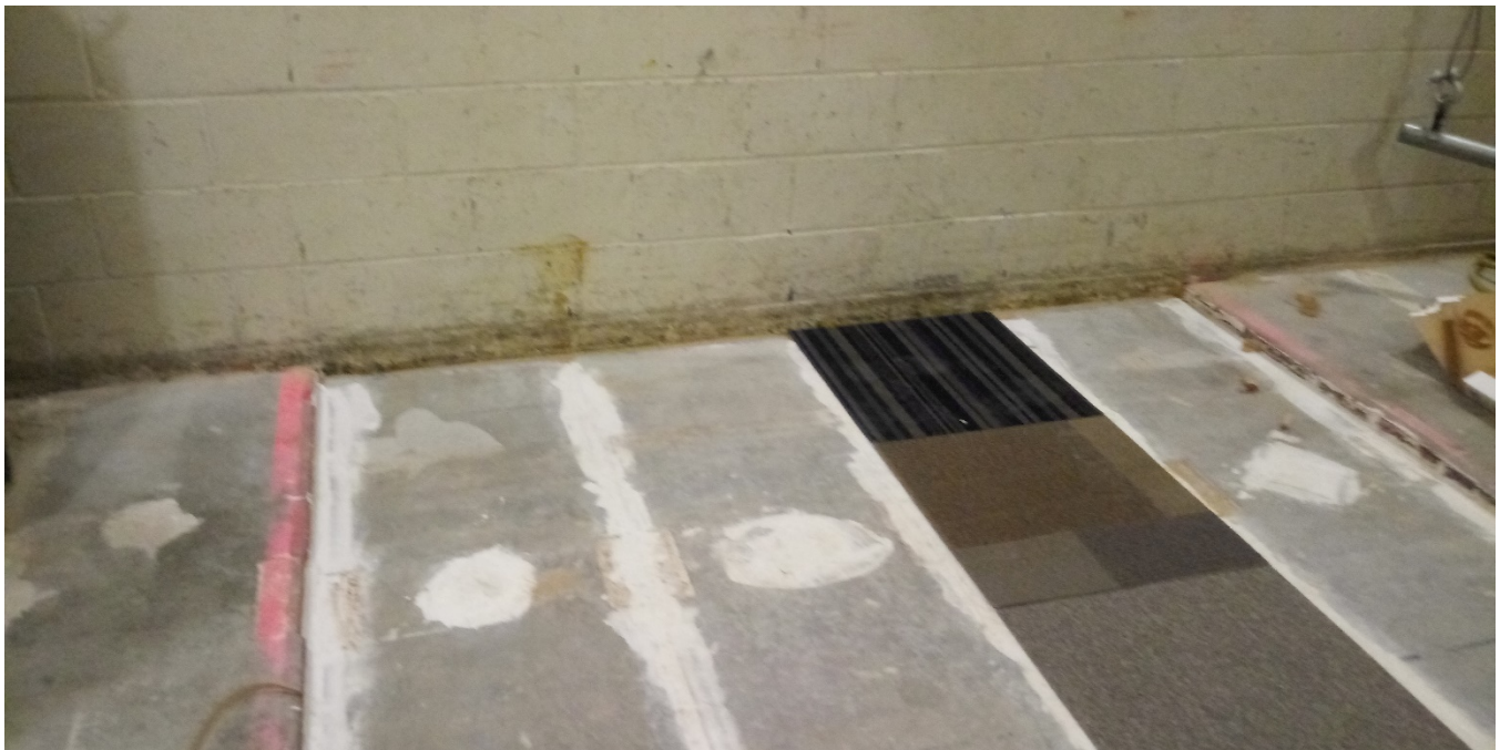
Figure 10 –Carpet flooring partially installed
