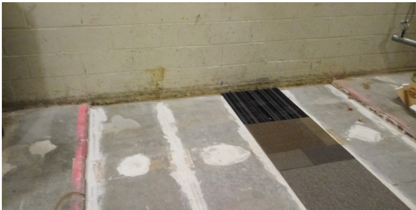
Figure 10 – Carpet tiles partially installed over concrete slabs
