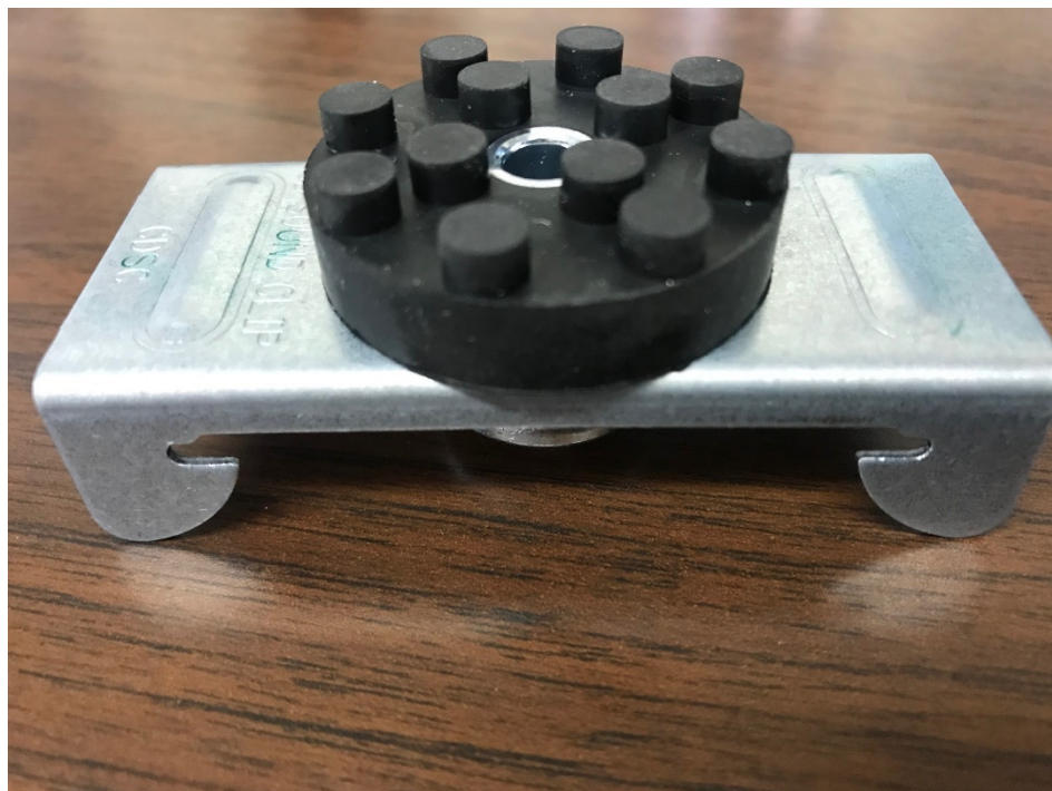
Figure 4 – Detail of isolating clip
