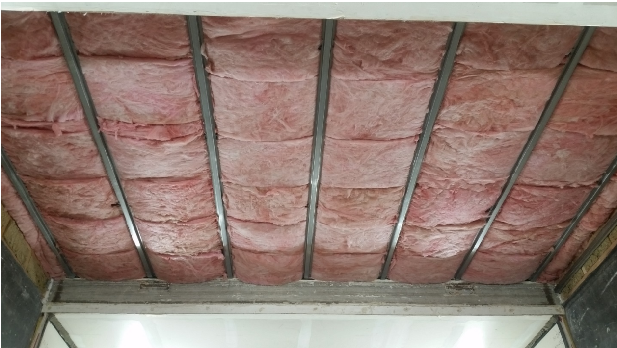
Figure 8 – Furring channel and insulation installed below slabs
