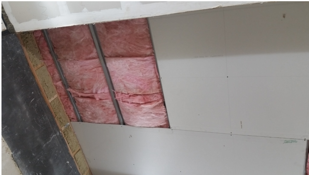
Figure 9 – Gypsum board partially installed to furring channel
