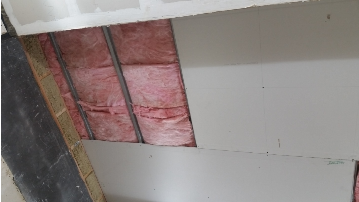
Figure 9 – Gypsum board partially installed to furring channel
