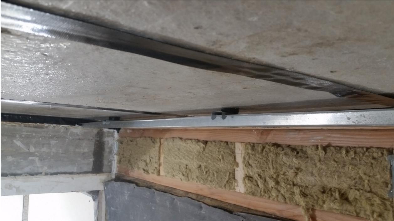
Figure 7 – Furring channel being installed to isolating clips
